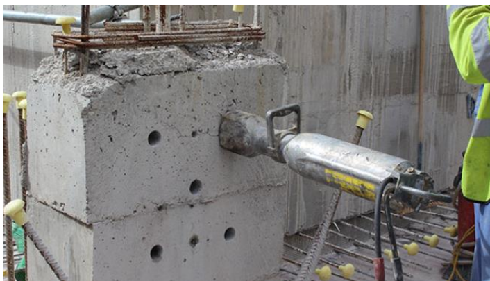
Figuur 33: Hydraulische splijtmachine (website Specialist Cutting Services Limited)
